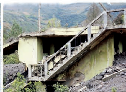
FIVE MISSING AFTER ROCKS AND MUD 4) ..... HOMES IN VILLAGE
