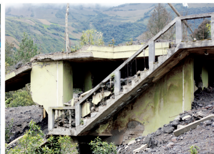
FIVE MISSING AFTER ROCKS AND MUD 4) ..... HOMES IN VILLAGE
